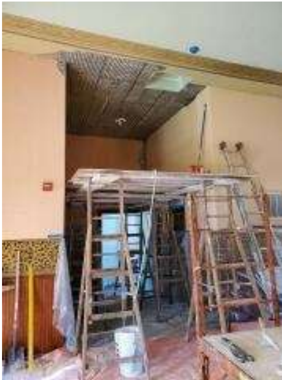
TOWN HOUSE PLASTER REPAIR
